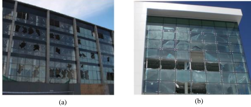
Figure 1. Glazing damage observed in past earthquakes (a) 2010 Chile earthquake (b) 2011 Christchurch earthquake.
